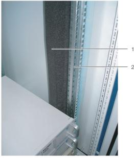
Fig. 15: Foam strip on a server rack upright
